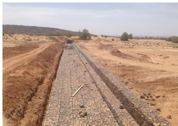
Photo n°2 : Gabion anchor ensuring the solidity of the work
